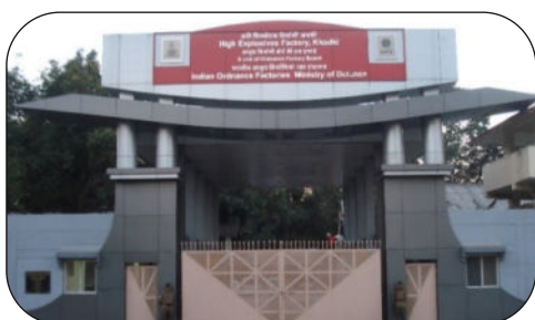
High Explosive Factory Khadki (HEF)
